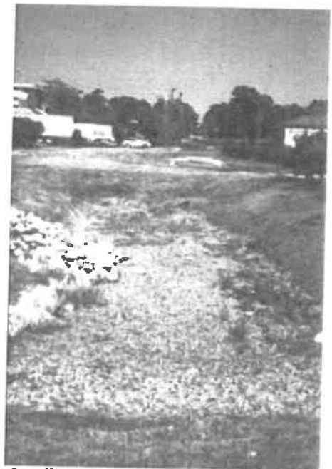
A well-maintained detention or dry pond.
