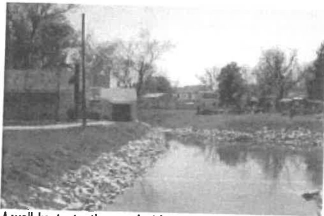
A well-kept retention pond with rip rap.
