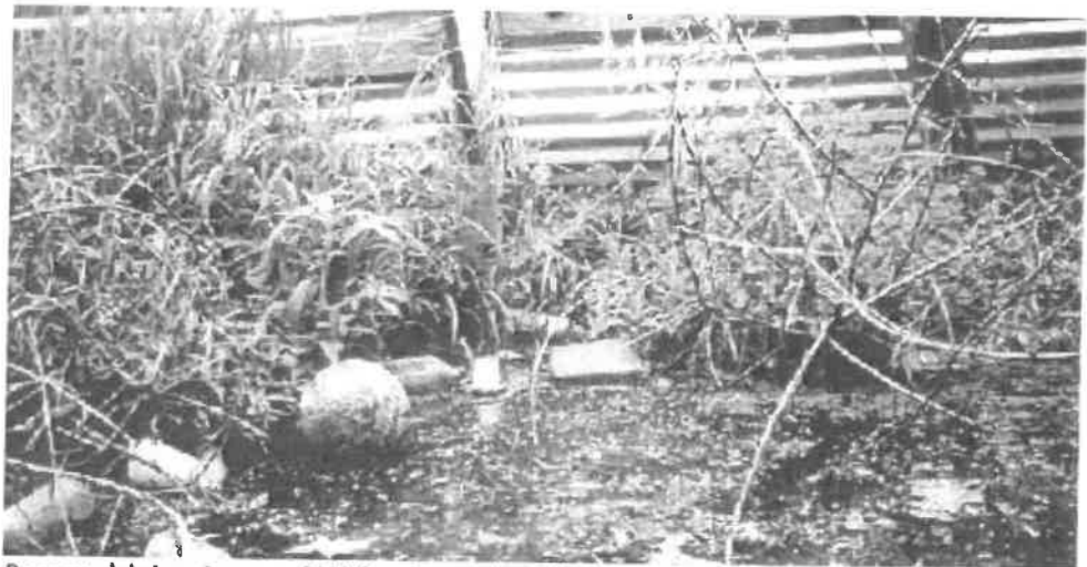
Remove debris to improve BMP function and aesthetics.
